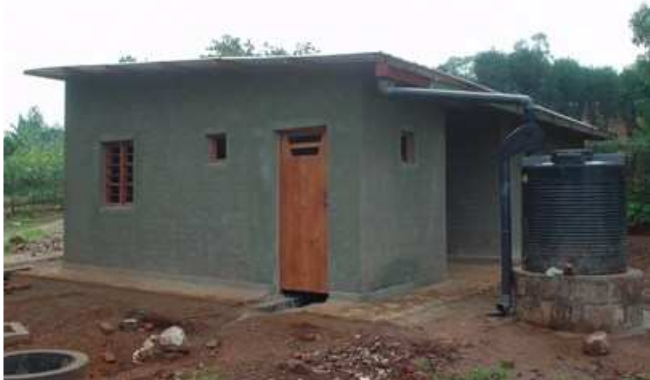
Typical housing unit in Batsinda
